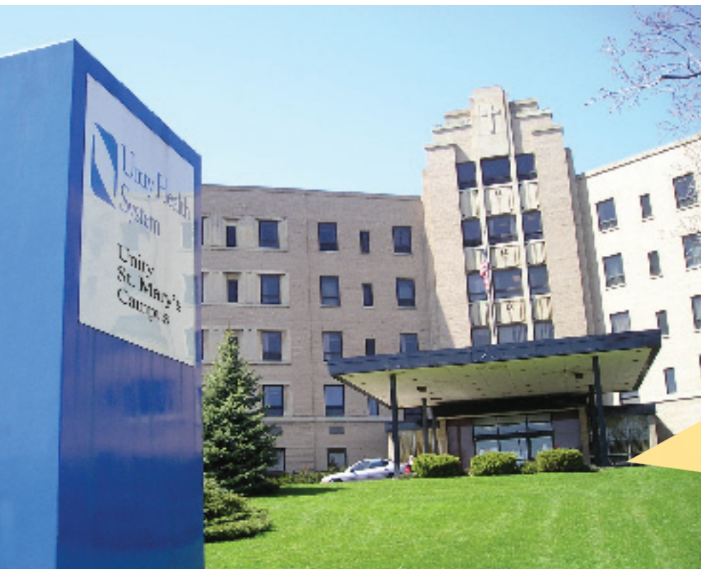
Unity St. Mary's Campus: A true multi-use facility, this health and human services center is the hub of numerous health and outreach services.
